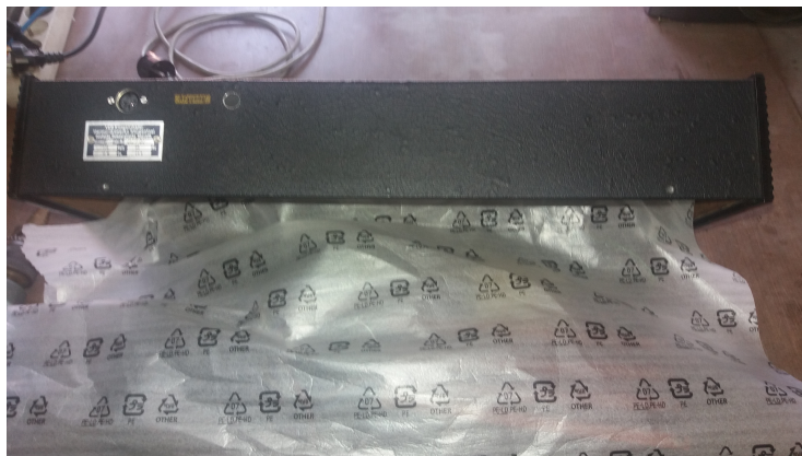
Figure 2: Covering electronics before drilling
